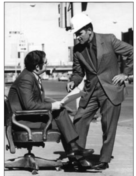
Joe Shocter during the construction phase of the Citadel Theatre, 1976. JAHSENA photo donated by the Shocter family.
